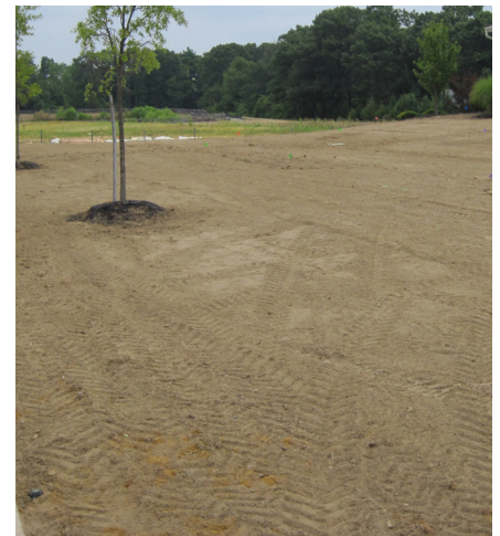
Graded soil in a home lawn area during lawn renovation.
